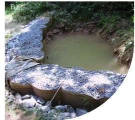
A. Stabilize Soil, Control Floods B. Control Erosion and Sediment Cellular Confinement Systems
