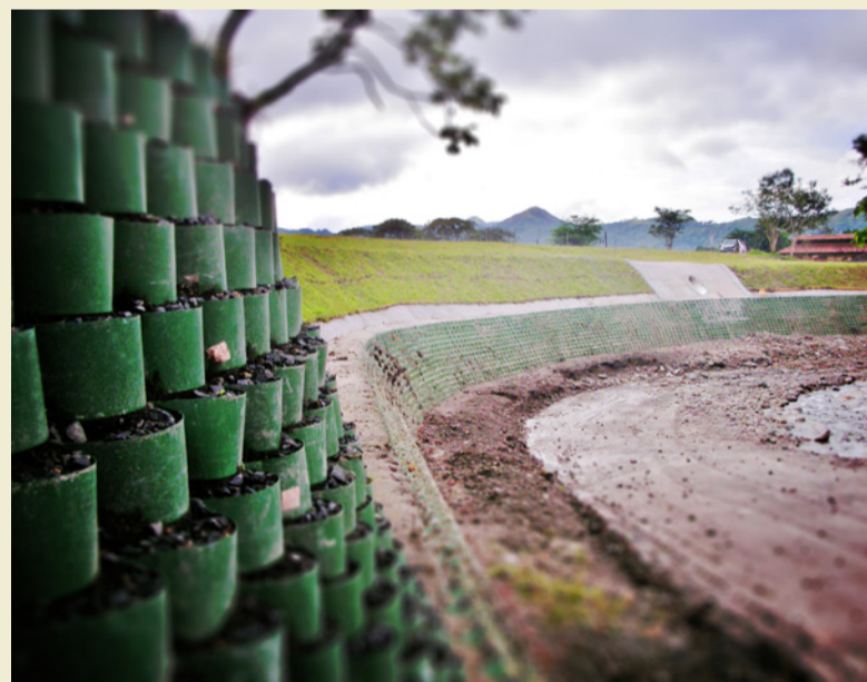
Los Portales, Rio Guayabo (Completed project)
