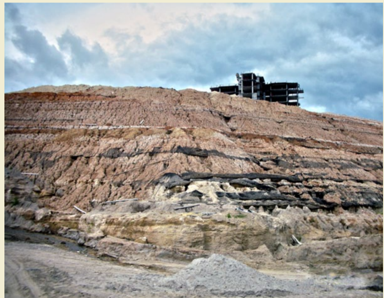
Bijao Beach Resort (Pre-Envirogrid Slope Erosion Control System)
