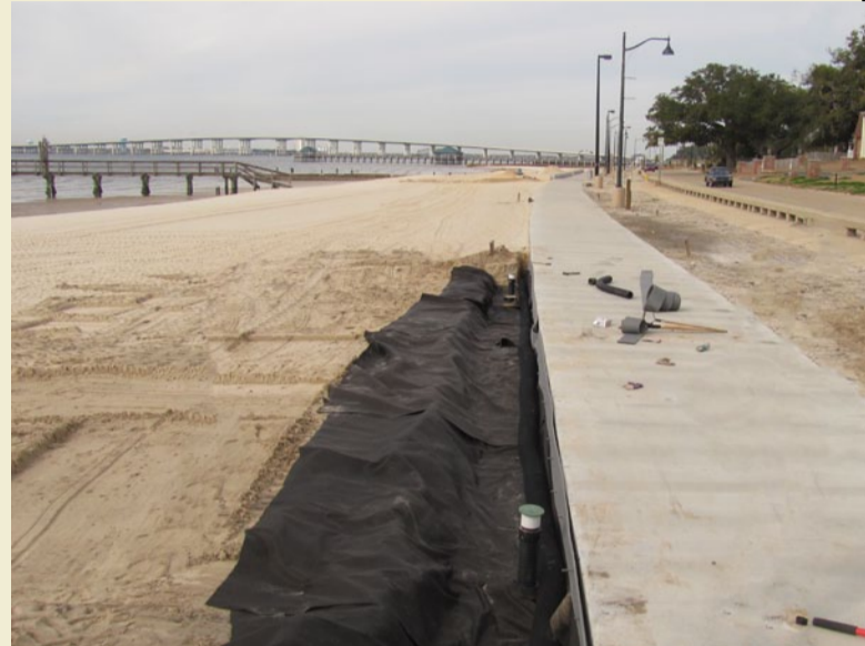
Ocean Springs Beach Sidewalk (Pre-Envirogrid Cellular Confinement System)
